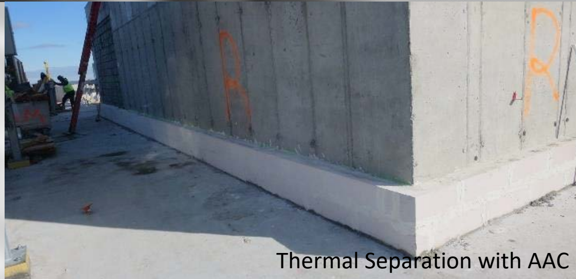
Thermal Separation at Dunnage
